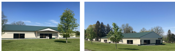
Finishing touches are being done on the new NY Conference Pavilion, just in time for campmeeting.
